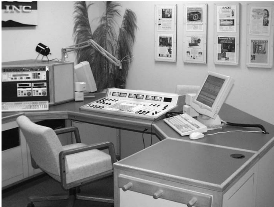
FIGURE 2.8 Any audio studio should be a comfortable and functional environment. (Image courtesy of Arrakis Systems, Inc. www.Arrakis-Systems.com .)
